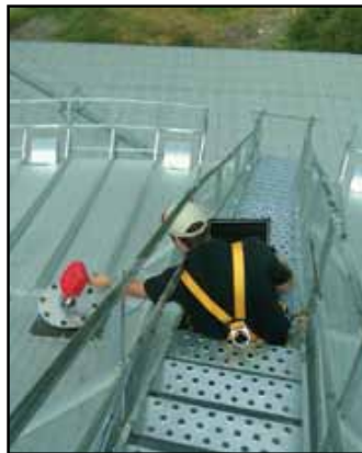
Most big bins have a single ladder from the sidewall to the peak for bin access.
